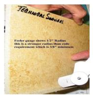
• The following illustrations show the basis of design for Sanitary Cove Base and a correct as well as incorrect installation profile. Setting Cove Base on top of the field tile is sometimes necessary though flush with floor tile as shown is recommended. *Regardless of installation method the joint where cove base meets floor should be treated as a perimeter joint and filled with flexible material instead of grout, per EJ*-*171 of the TCNA Handbook.*
